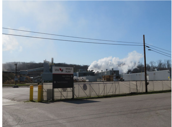
Figure 3.24-6 Gypsum Processing Plant and Mine East of Shoals, Martin County, north of US 50.
