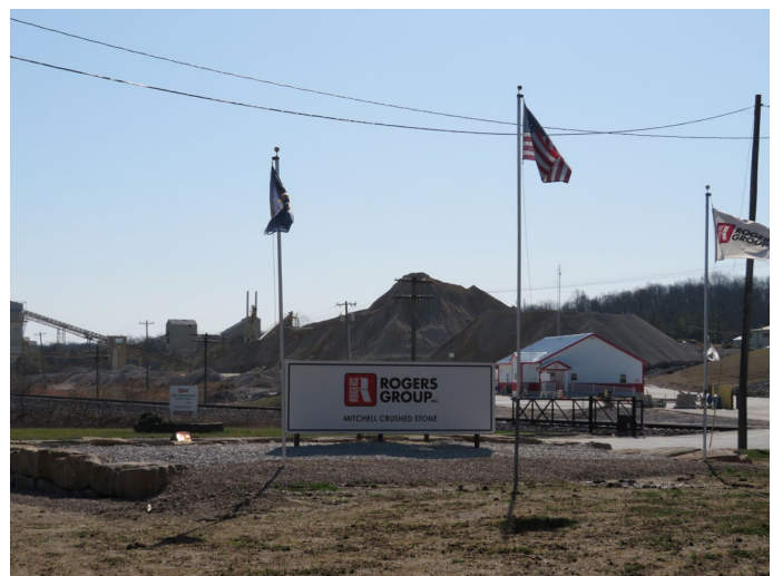
Figure 3.24-5 Limestone Quarry Operation at the Village of Georgia on SR 60
