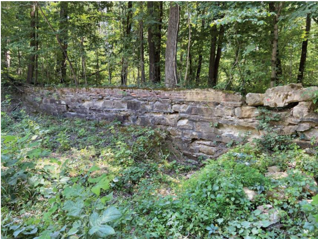
Photo ID 604, Stone and Brick Wall, CR 500 S, Corning; Alternative C
