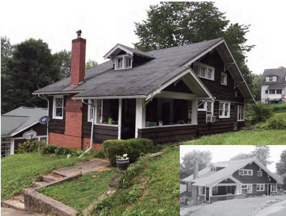
Photo ID 952, House, Ballard Homes Historic District, potentially NRHP-eligible, French Lick; Alternative O
