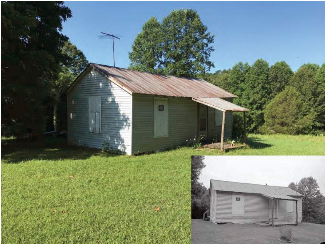
Photo ID 1045, House, CR 610 N, Orange Co.; Alternative O
