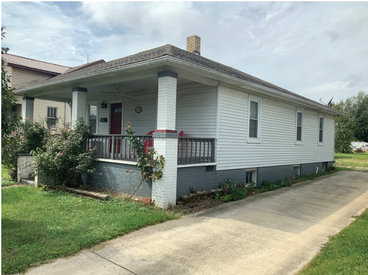
Photo ID 3196, House, 1106 N. Main Street, Huntingburg; Alternative R
