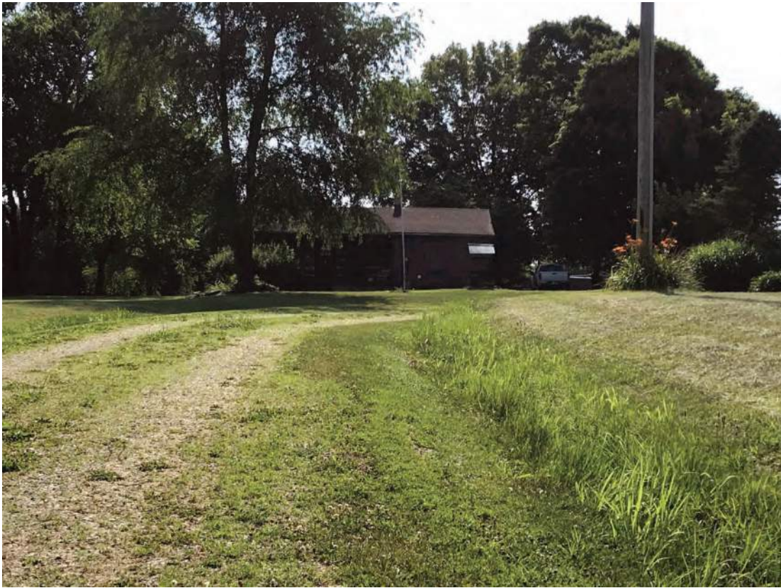
Photo ID 372, Log House, potentially NRHP-eligible, 8210 S 200 W, Dubois Co.; Alternatives M, O, P
