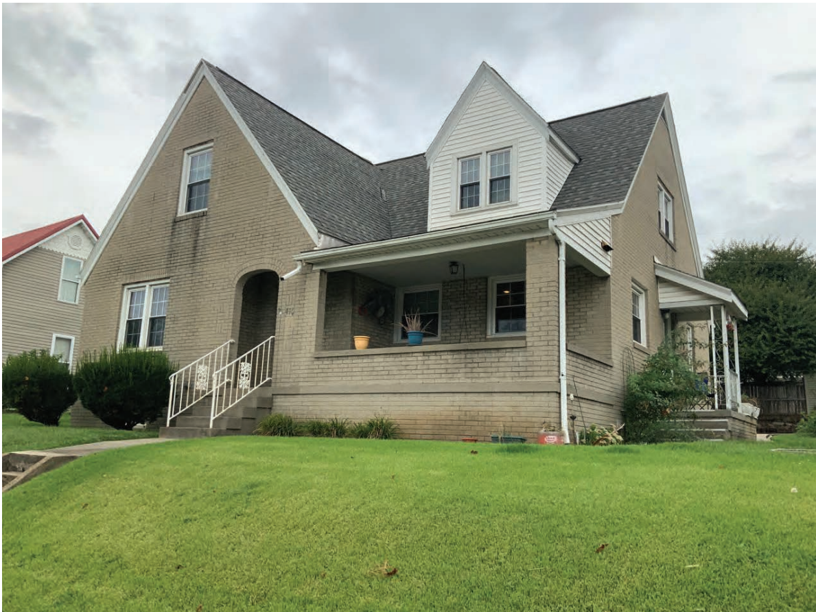
Photo ID 1899, Jasper Residential Historic District #1, potentially NRHP-eligible, 416 W. 6th Street, Jasper; Local Improvement 4
