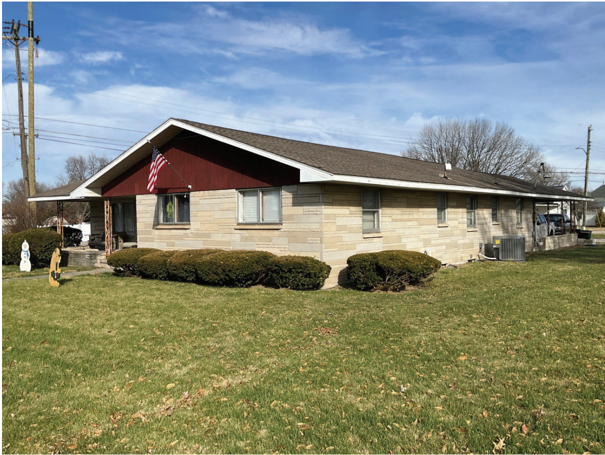
Photo ID 2167, House, 501 John F. Kennedy Avenue, Loogootee; Alternative P2
