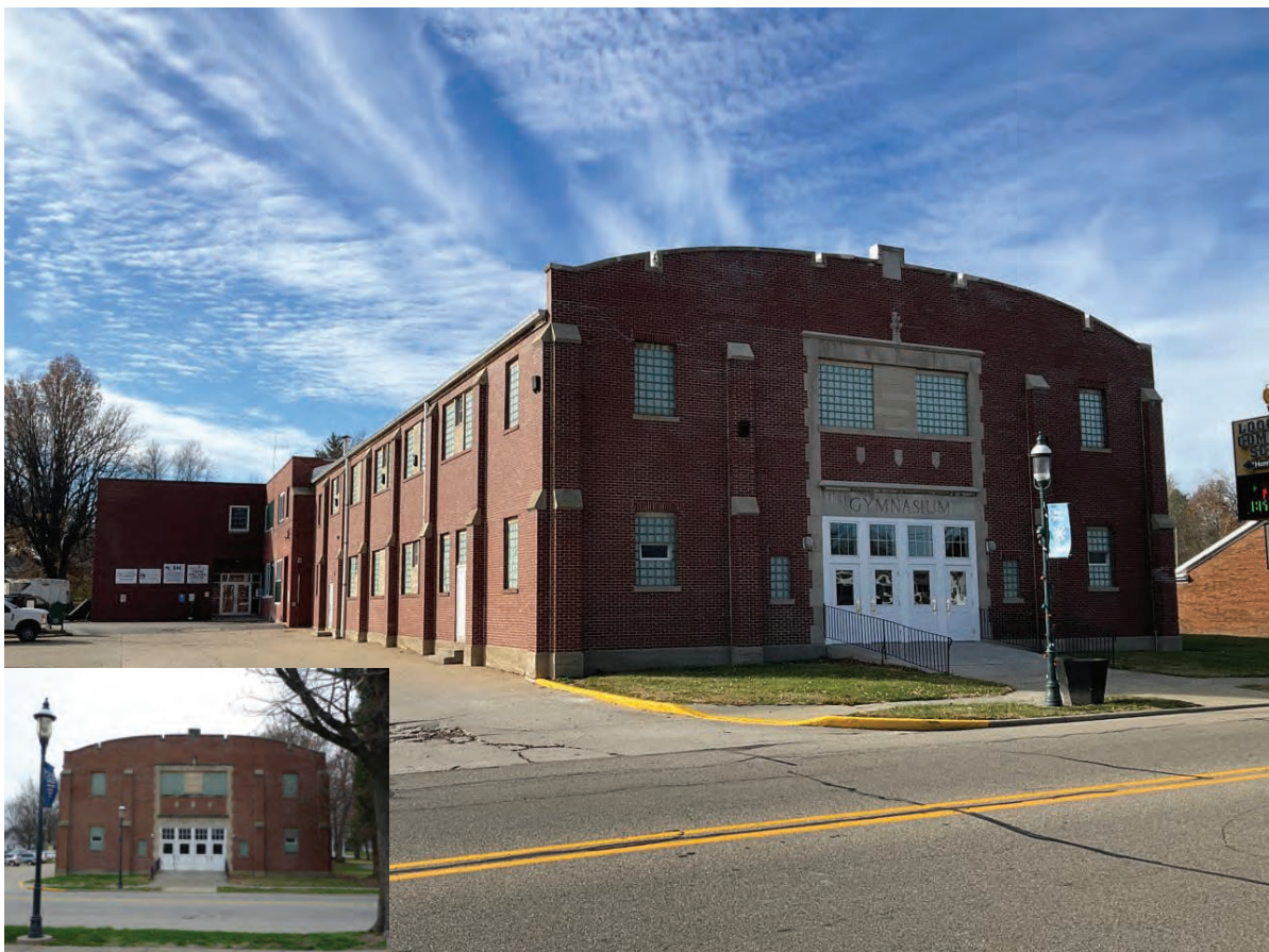
Photo ID 2164, NRHP-eligible, Loogootee Gymnasium, 405 N. John F. Kennedy Avenue, Loogootee; Alternative P2
