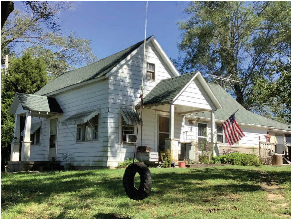
Photo ID 2032, House, 4234 N SR 257, Otwell; Local Improvement 11
