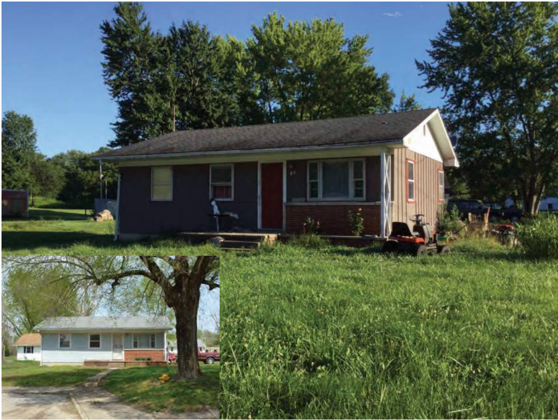
Photo ID 1530, House, Crane Historic District, potentially NRHP-eligible, Crane; Alternative P
