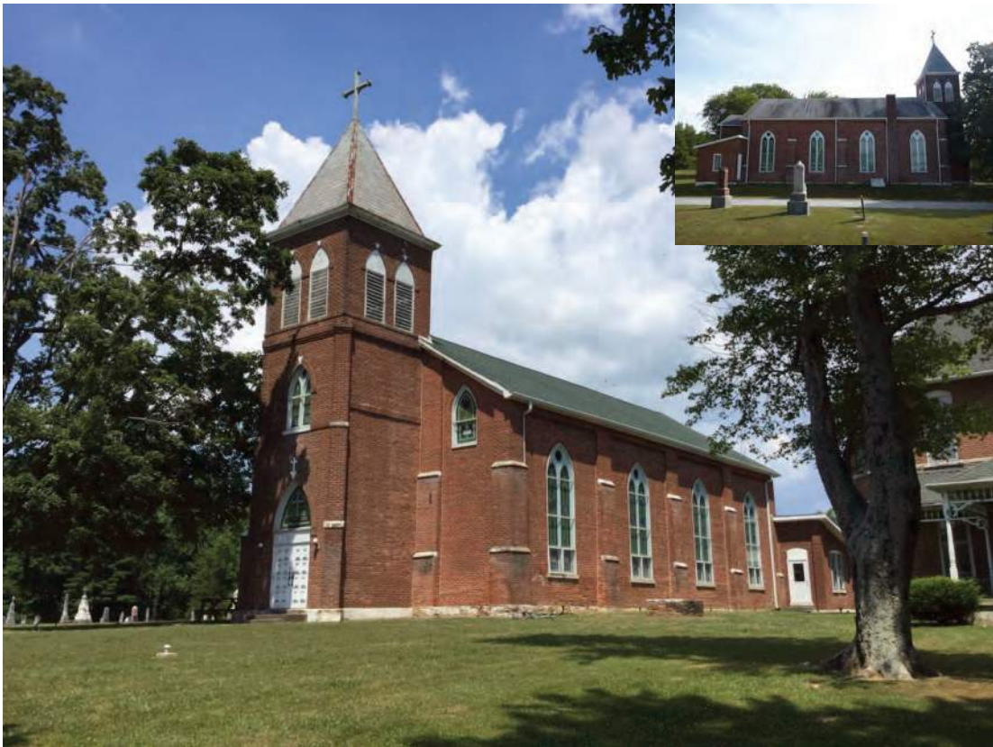
Photo ID 596, Saint Patrick's Catholic Church, potentially NRHP-eligible, 4962 S 800 E, Daviess Co.; Alternative C
