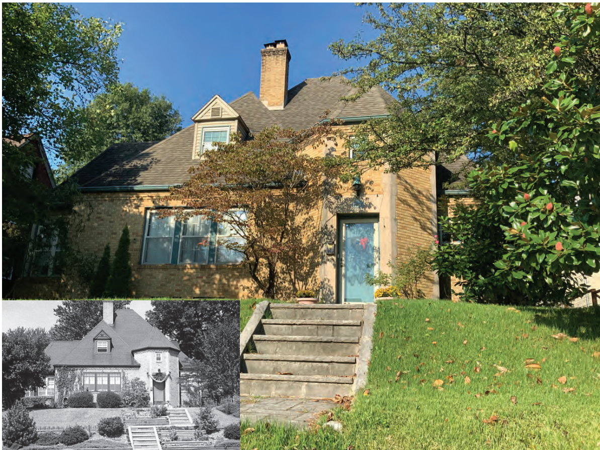
Photo ID 1968, Jasper Residential Historic District #2, potentially NRHP-eligible, Wilson House, 1431 Newton Street, Jasper; Local Improvement 4
