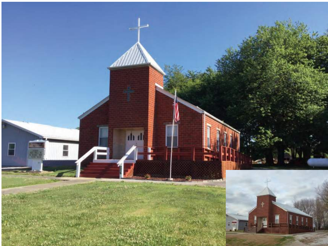
Photo ID 289, Hudsonville United Methodist Church, CR 825 S, Hudsonville; Alternative B
