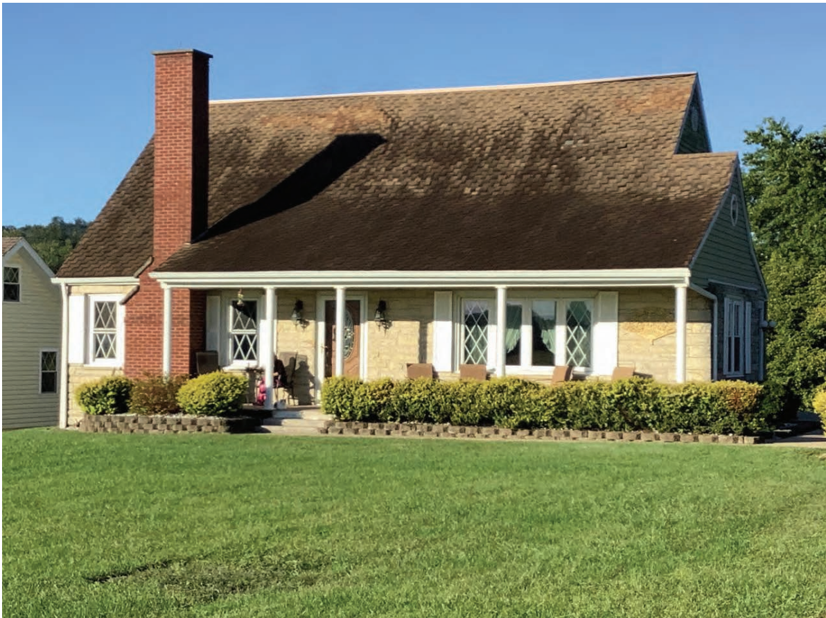
Photo ID 2093, House, 1377 N. Main Street, Prospect; Local Improvement 18
