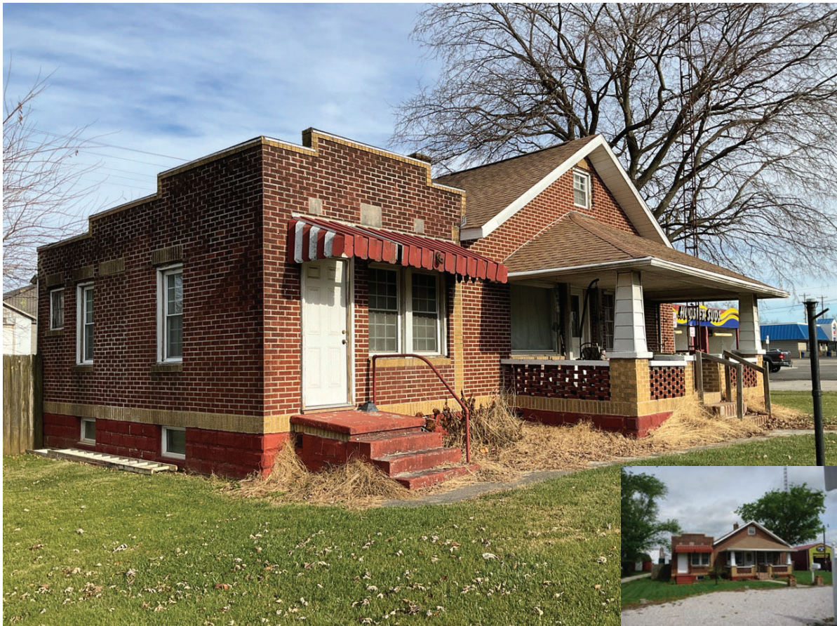
Photo ID 2146, House/Commercial Building, Contributing, 105 W. Broadway Street, Loogootee; Alternative P2
