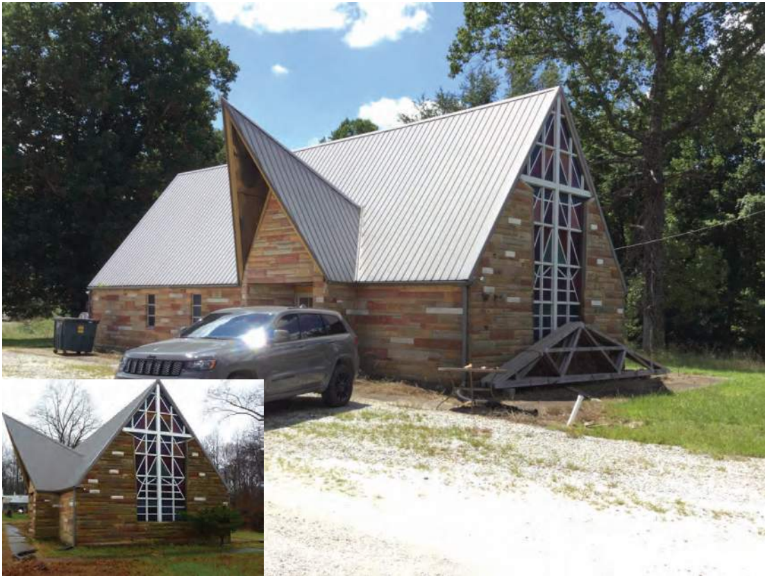
Photo ID 1389, Brinegar Chapel, potentially NRHP-eligible, 15955 N US Highway 231, Odon; Alternative P
