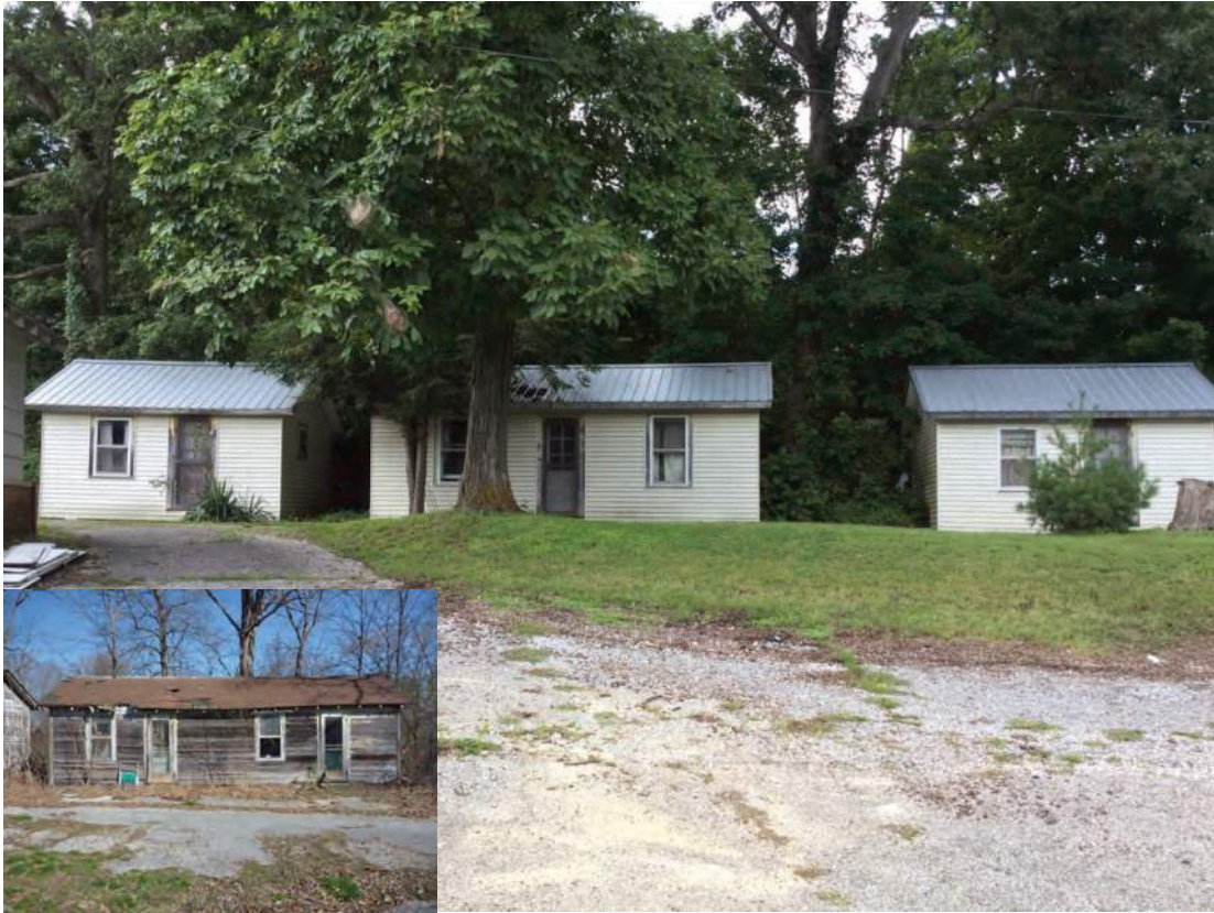
Photo ID 1340, Shady Nook Motel, potentially NRHP-eligible, 2083 US Highway 50, Martin Co.; Alternatives M, P
