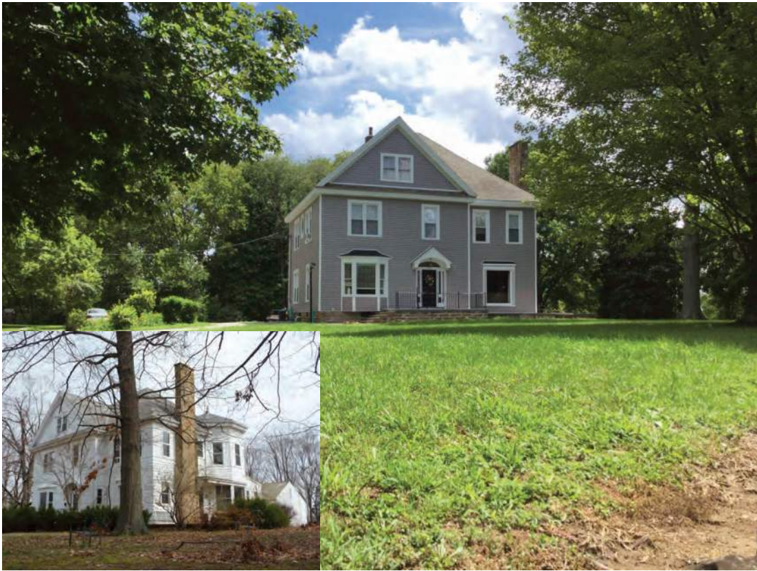
Photo ID 1252, Lewis c. Brooks House, potentially NRHP-eligible, 612 Kentucky Avenue, Loogootee; Alternatives M, P
