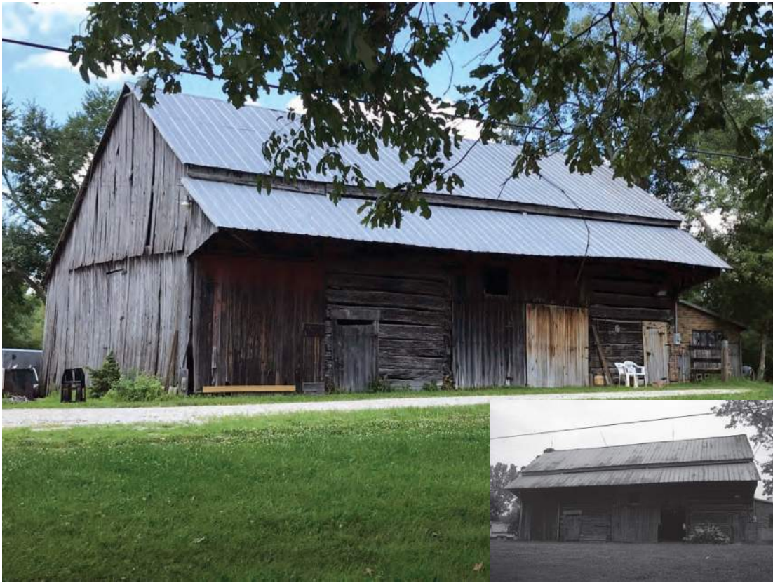
Photo ID 1477/1478, Schroeder-Fleck Log Barn, potentially NRHP-eligible, E. SR 164, Jasper; Alternatives M, O, P
