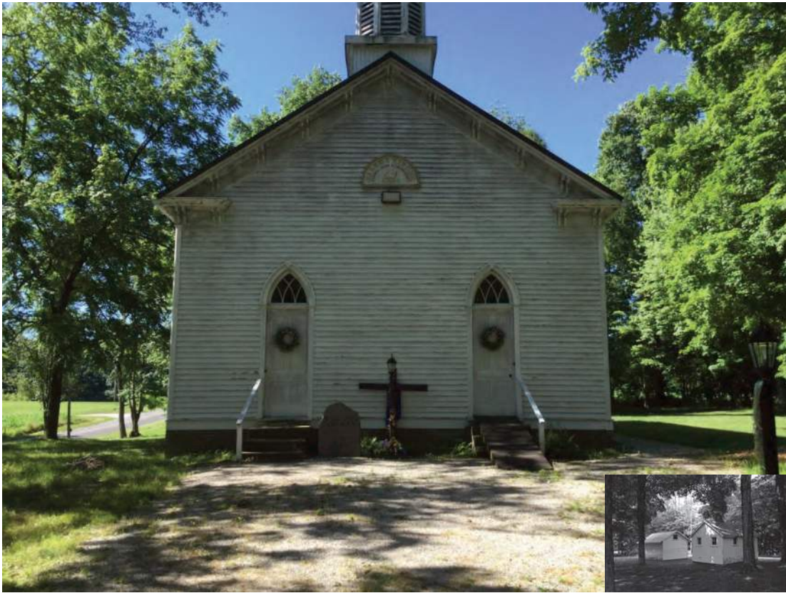
Photo ID 55, Maple Grove Methodist Campground, potentially NRHP-eligible, CR 585 W, Dubois Co.; Alternatives B, C
