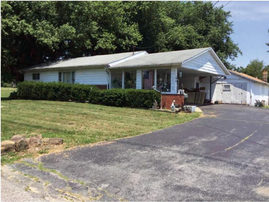
Photo ID 398, House, 250 E 100 S, Washington; Alternative B
