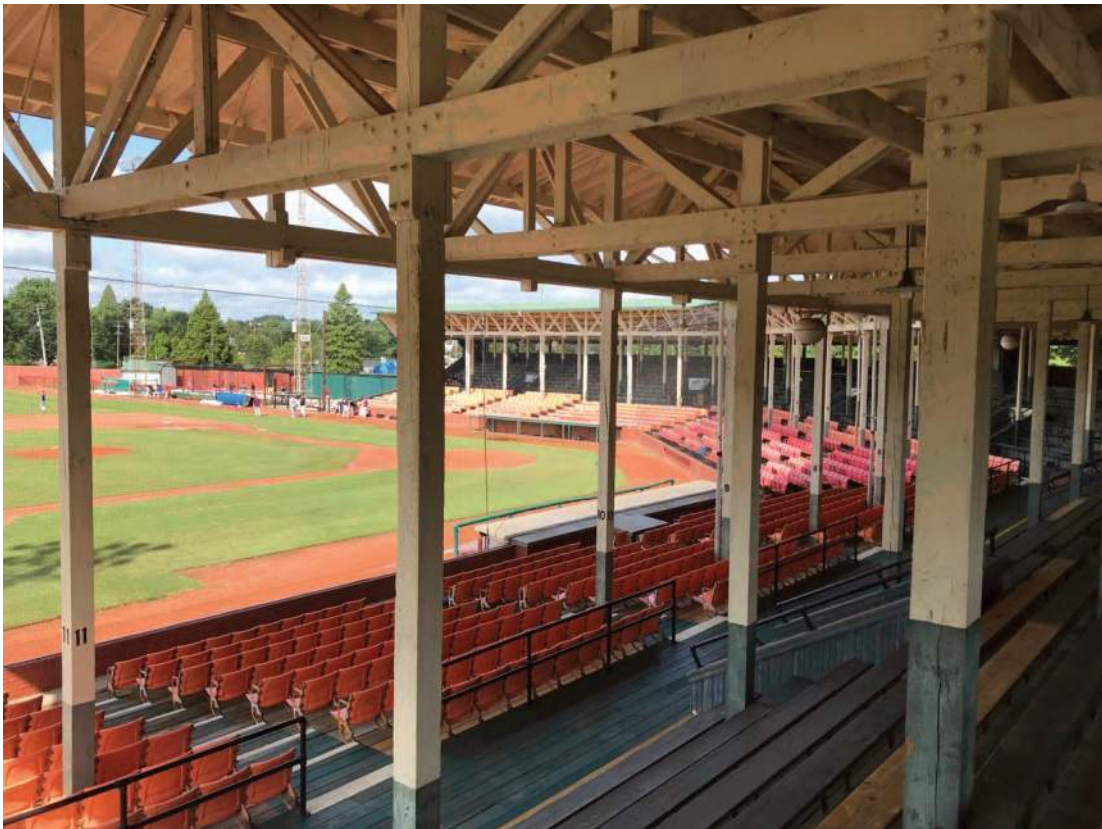
Photo ID 1179, League Stadium, potentially NRHP-eligible, 203 S. Cherry Street, Huntingburg; Alternatives M, P
