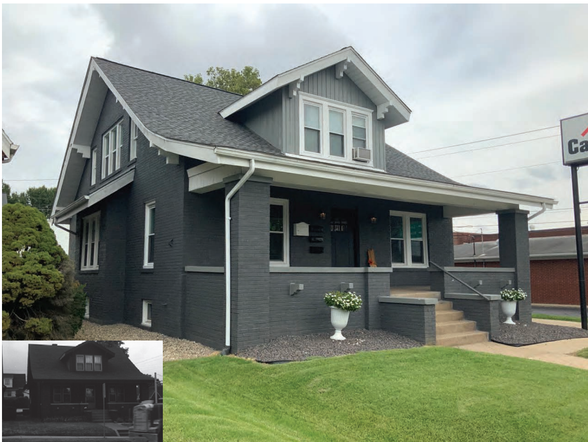
Photo ID 1905, Jasper Residential Historic District #1, potentially NRHP-eligible, 308 W. 6th Street, Jasper; Local Improvement 4
