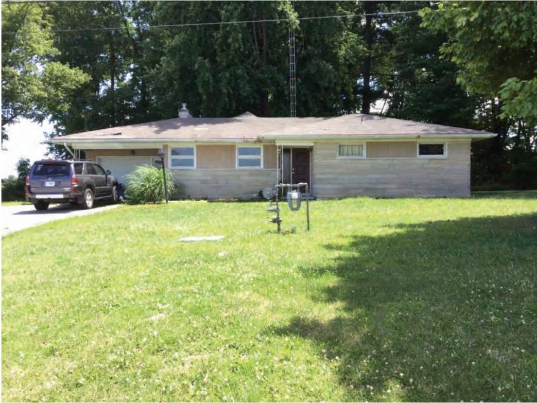
Photo ID 720, House, 2523 E National Highway, Washington; Alternative C
