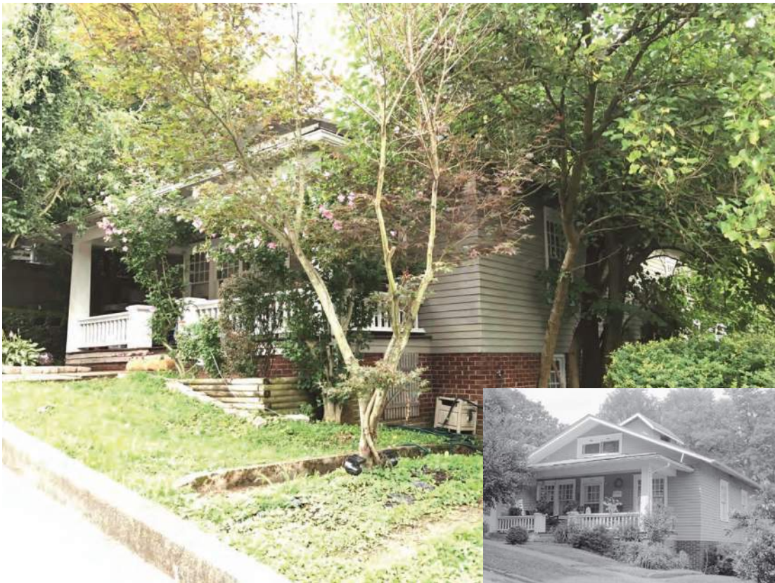
Photo ID 948, House, Ballard Homes Historic District, potentially NRHP-eligible, French Lick; Alternative O
