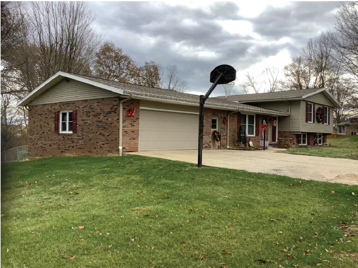
Photo ID 2212, House, 113 Crestview Drive, Loogootee; Alternative P3
