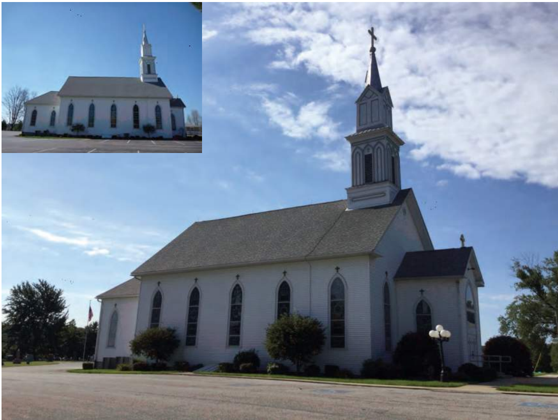
Photo ID 1353, Saint Joseph's Catholic Church, potentially NRHP-eligible, 18982 Saint Joseph Road, Martin Co., Alternative P
