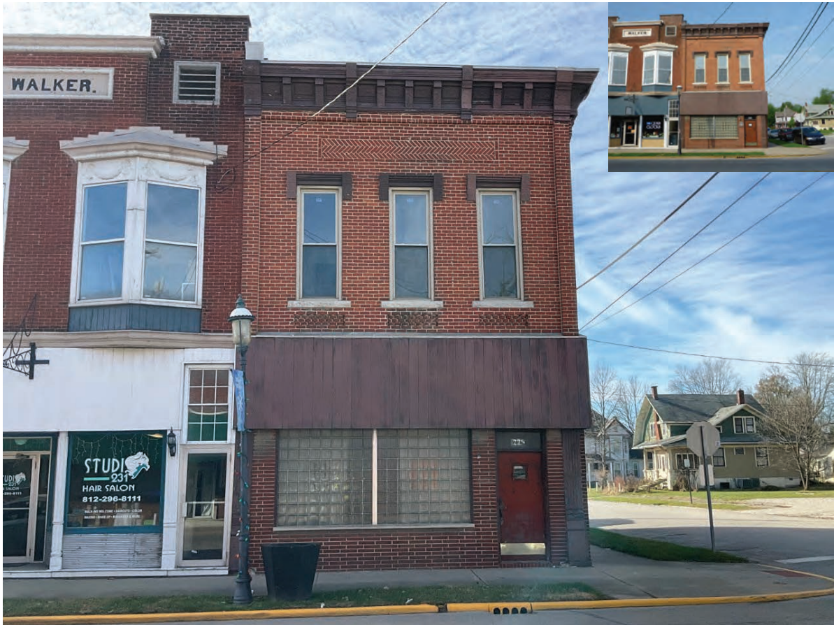
Photo ID 2161, Loogootee Commercial Historic District, NRHP-eligible, J.E. Porter/Jeweler Building, 229 N. John F. Kennedy Avenue, Loogootee; Alternative P2
