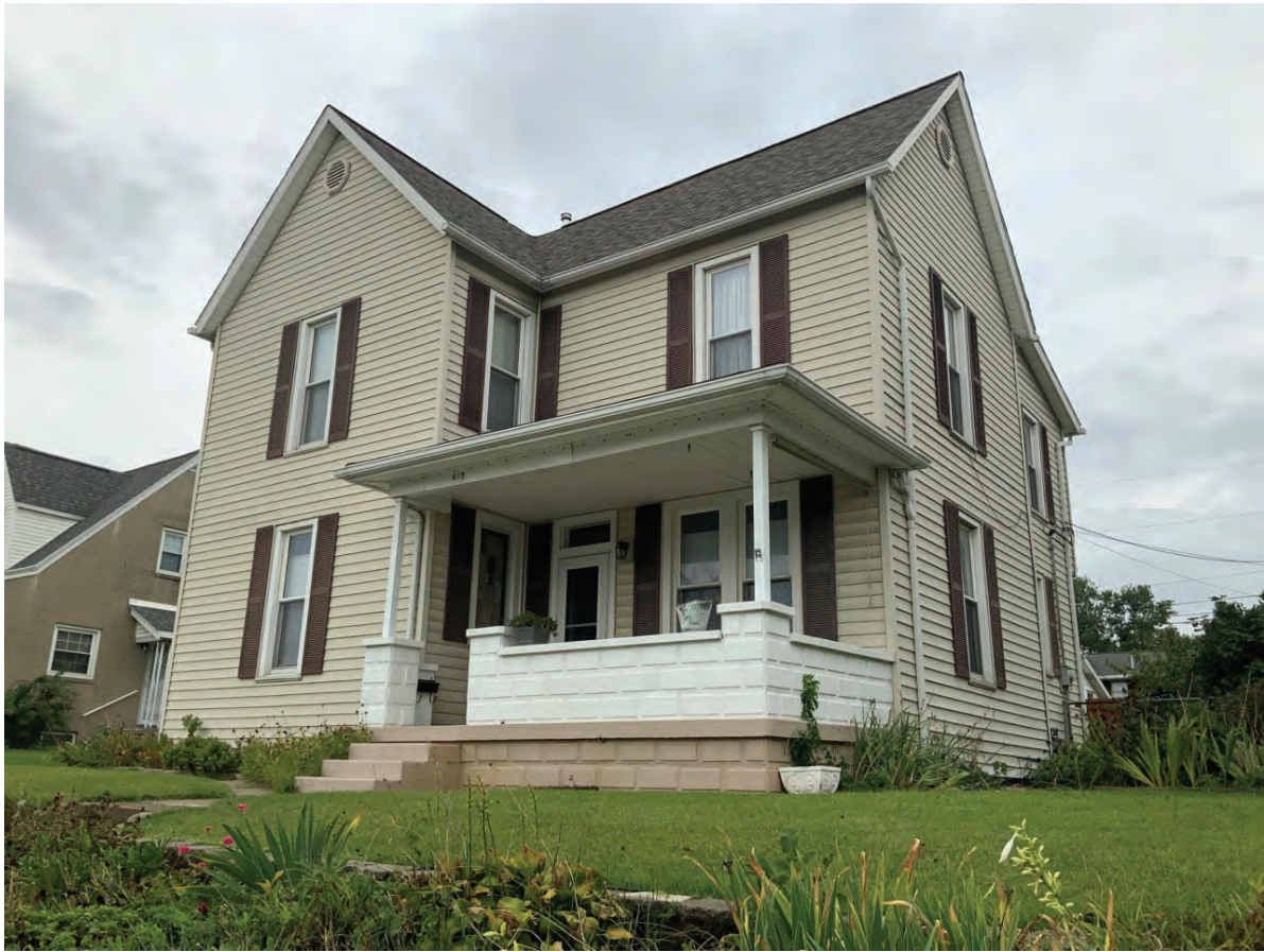
Photo ID 1900, Jasper Residential Historic District #1, potentially NRHP-eligible, 412 W. 6th Street, Jasper; Local Improvement 4
