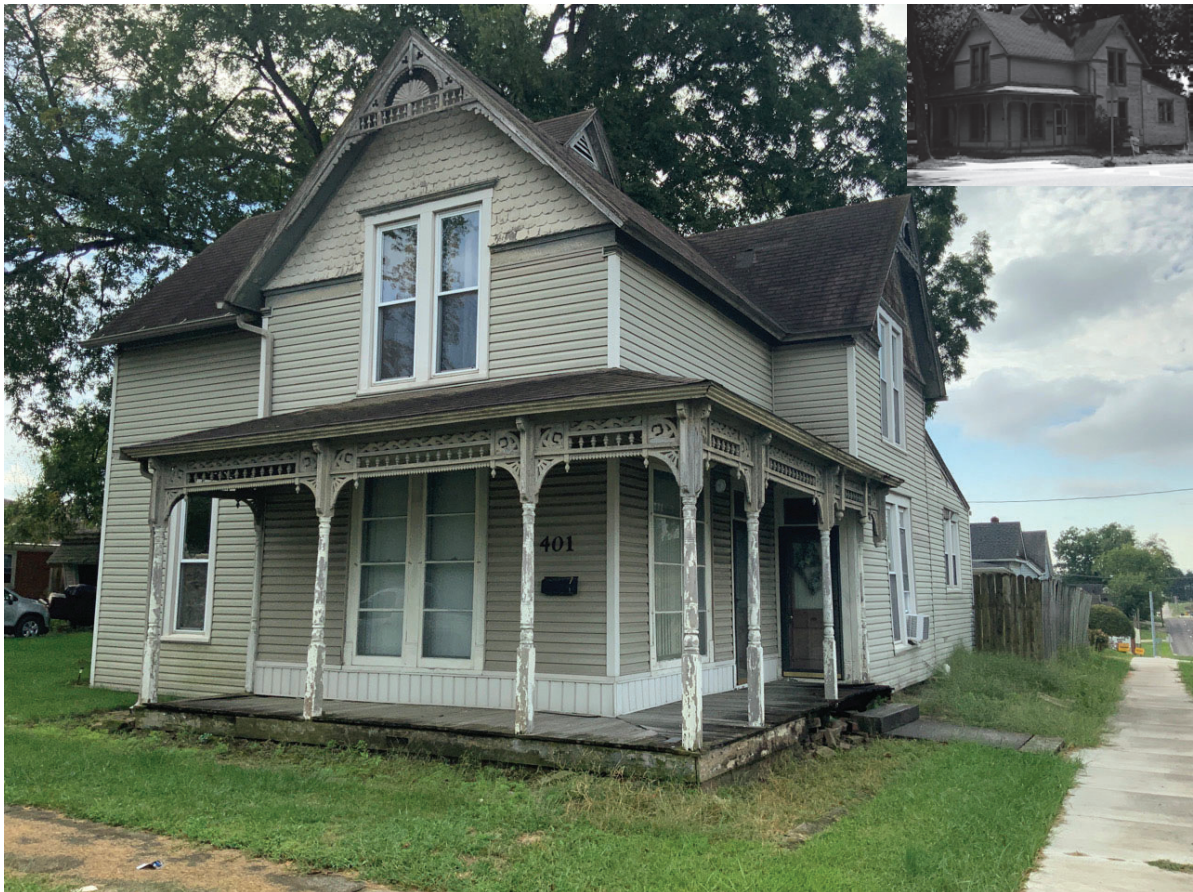
Photo ID 3185, House, Huntingburg Residential Historic District, 401 E. 2nd Street, Huntingburg; Alternative R
