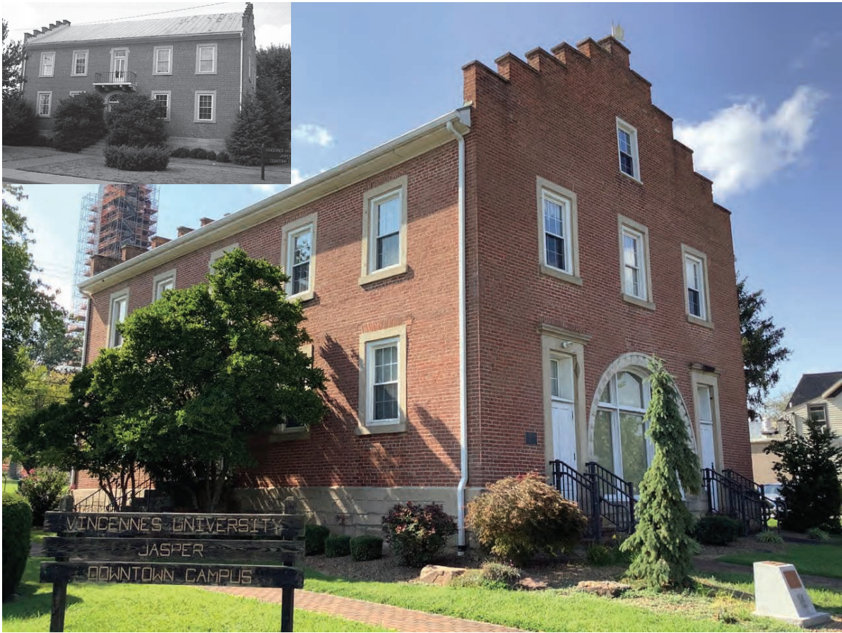
Photo ID 2129, Gramelspacher-Gutzweiler House, NRHP-listed, 1103 Main Street, Jasper; Local Improvement 4
