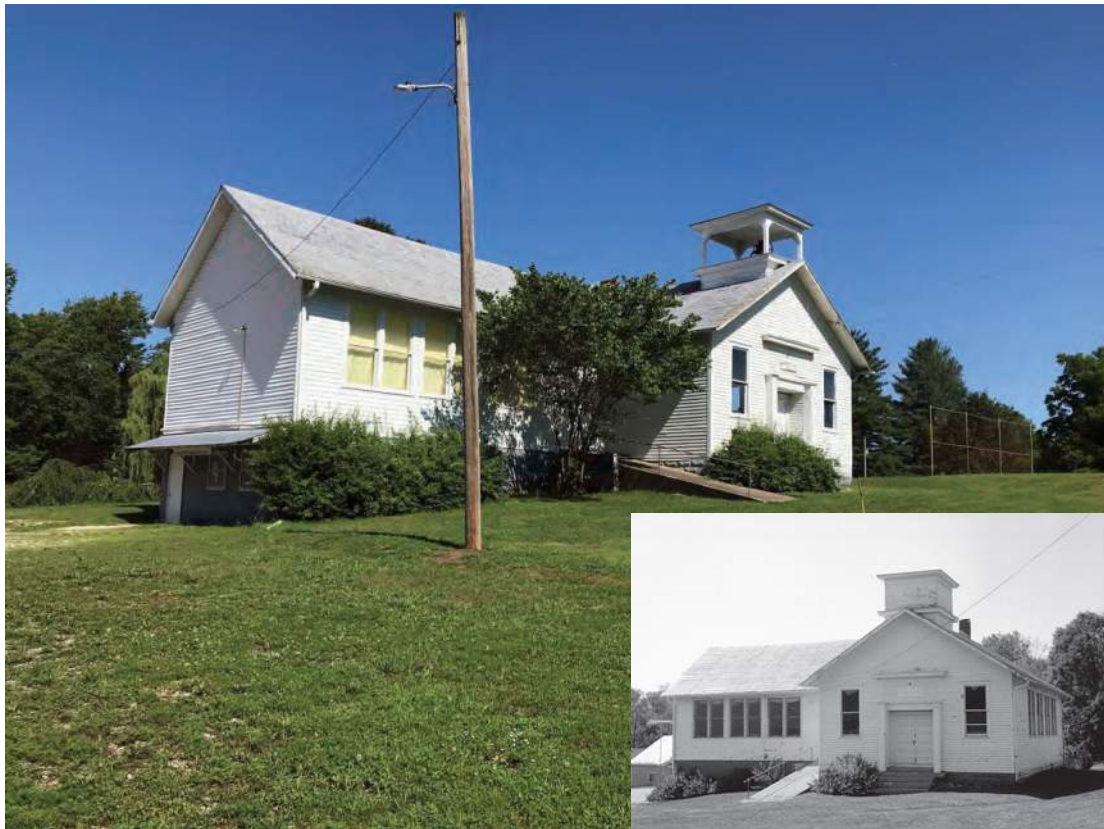
Photo ID 1056, Orangeville School, potentially NRHP-eligible, 5155 N 500 W, Orleans; Alternative O
