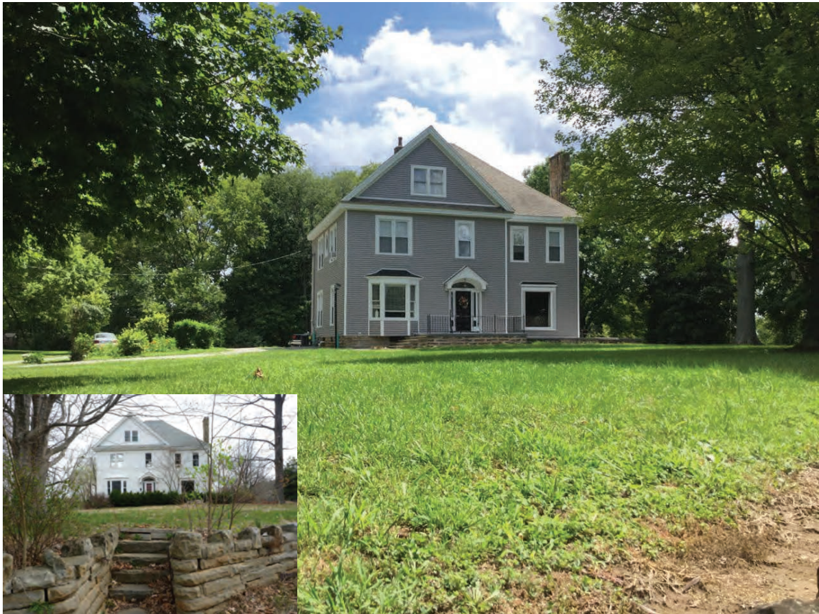
Photo ID 1252, NRHP-eligible, Lewis C. Brooks House, 612 Kentucky Avenue, Loogootee; Alternative P3
