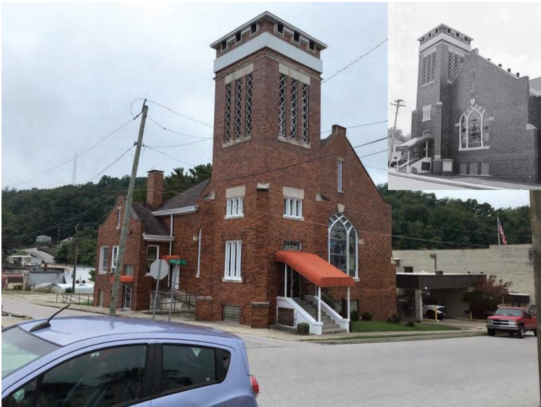
Photo ID 938, Springs Valley United Methodist Church, potentially NRHP-eligible, 537 S. Maple Street, French Lick; Alternative O
