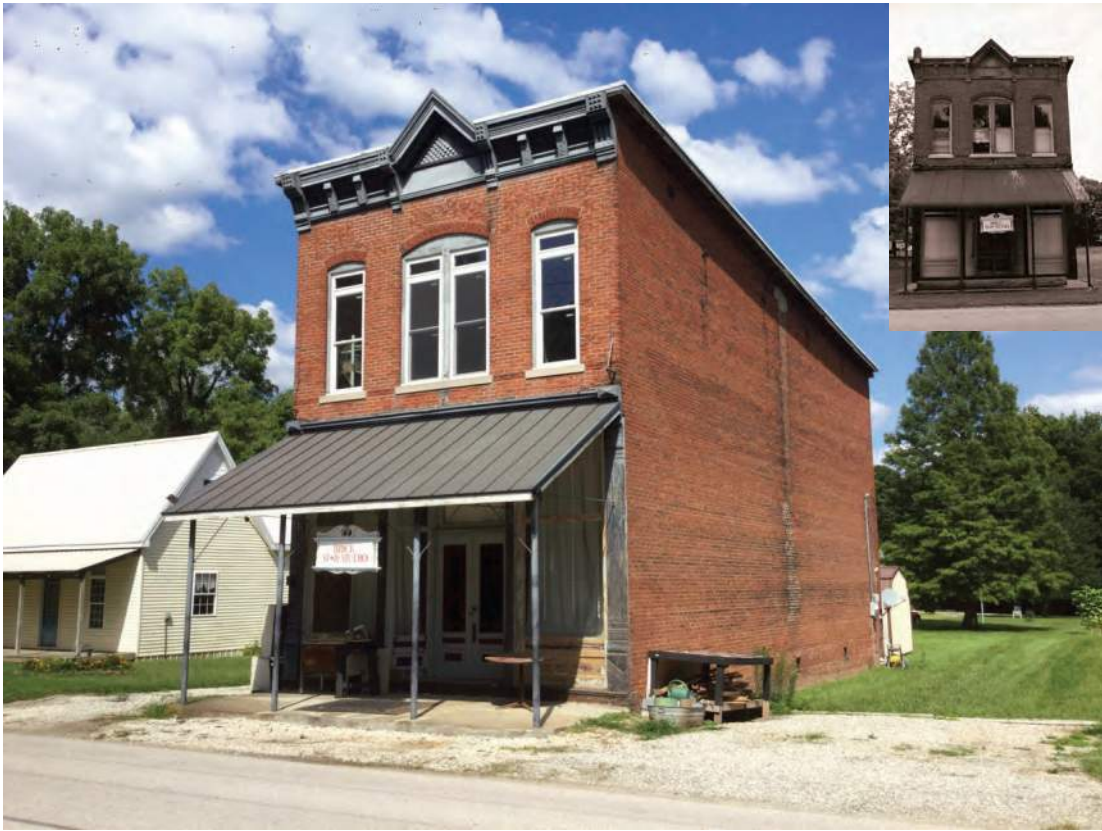
Photo ID 1425, Blackmore Store, potentially NRHP-eligible, Main Street, Scotland; Alternative P
