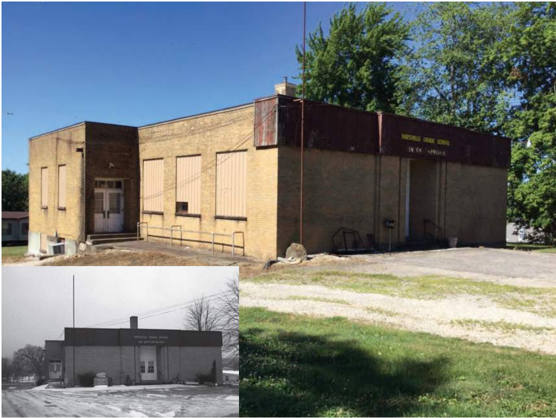
Photo ID 682, Haysville Grade School, 352 W. Haysville Road, Haysville; Alternatives C, M, P
