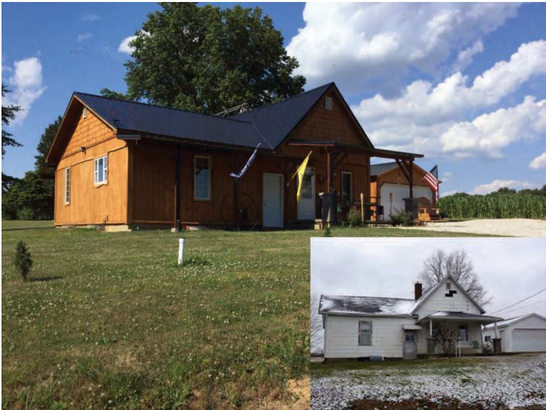
Photo ID 353, House, 1782 E 300 S, Daviess Co.; Alternative B
