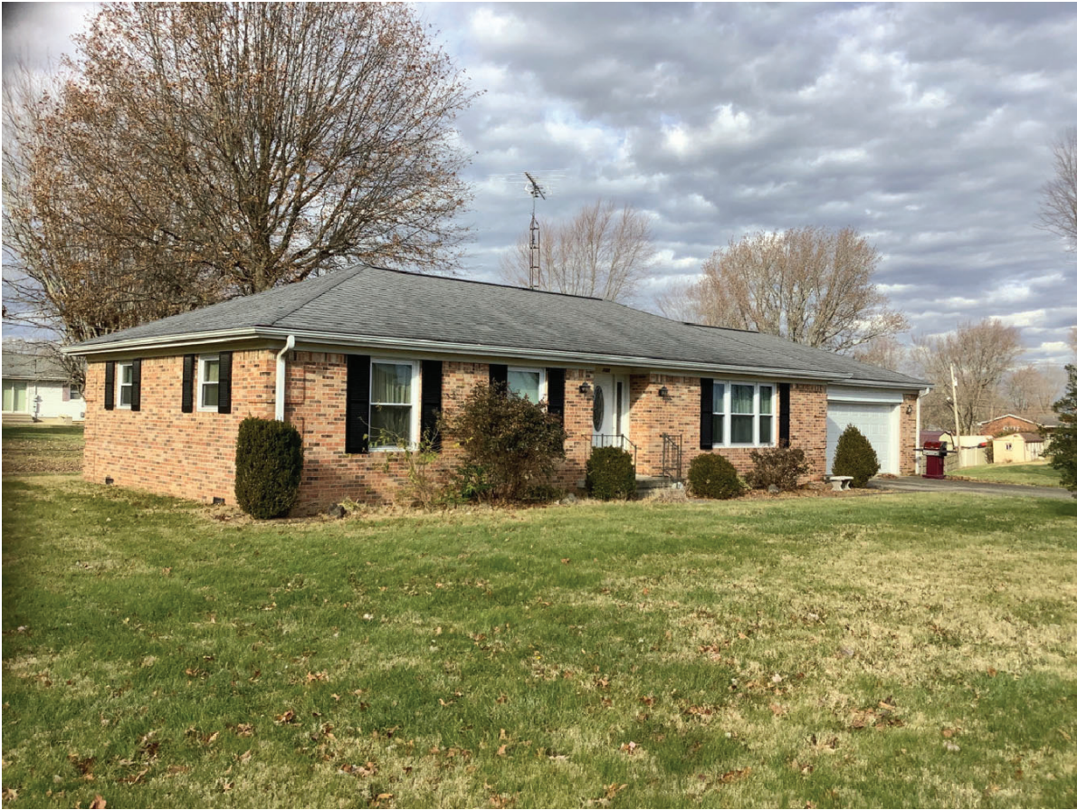
Photo ID 2206, House, 100 Crestview Drive, Loogootee; Alternative P3
