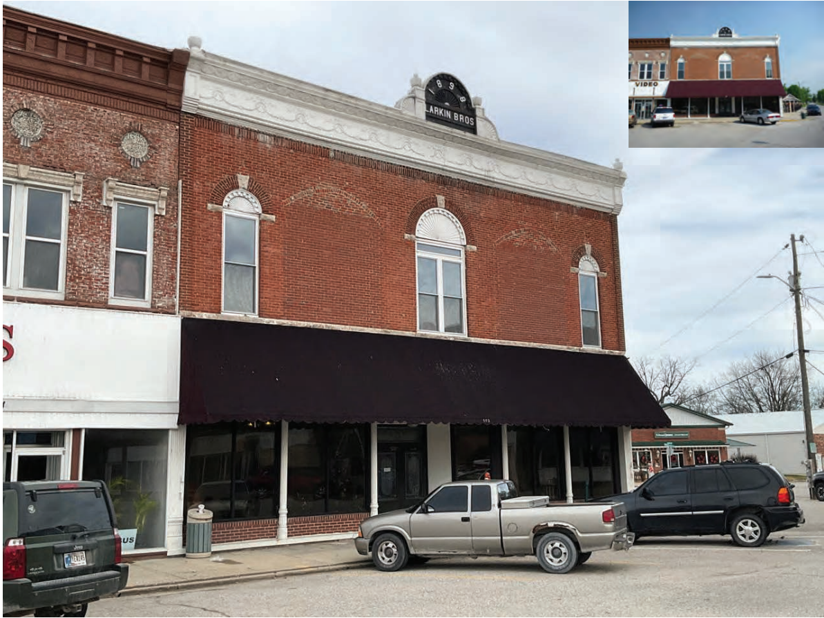
Photo ID 2157, Loogootee Commercial Historic District, NRHP-eligible, Larkin Bros. Building, 103 Wood Street, Loogootee; Alternative P2
