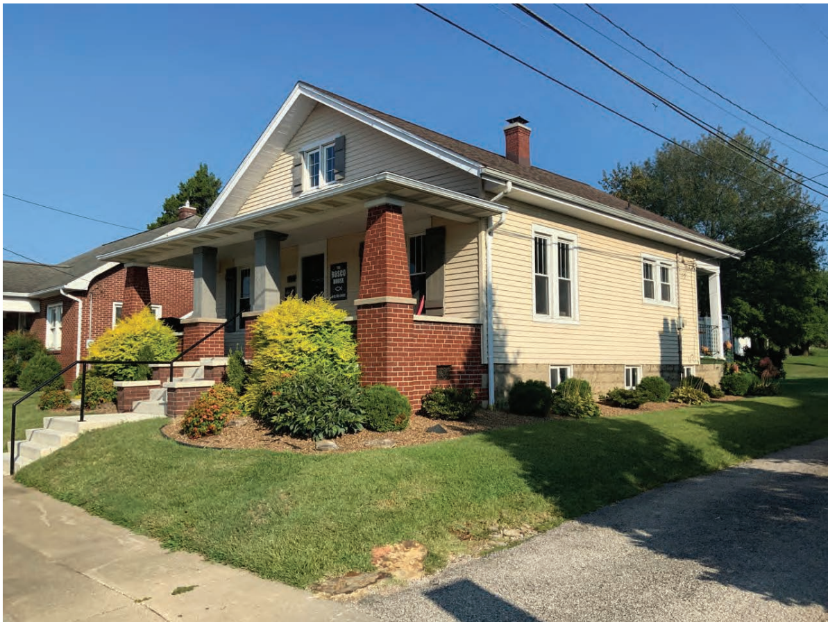
Photo ID 1957, House, 214 W. 13th Street, Jasper; Local Improvement 4
