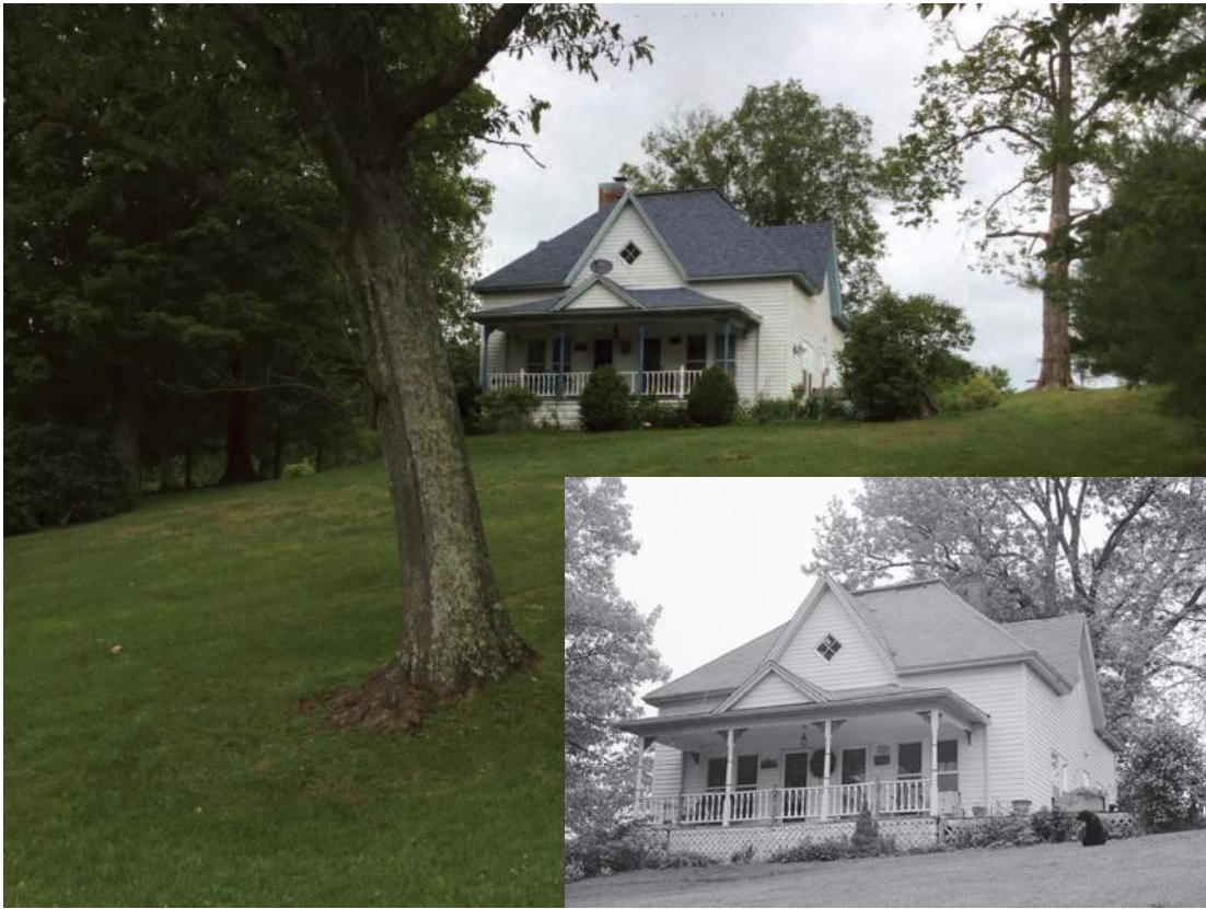
Photo ID 904, George Campbell House, potentially NRHP-eligible, 6284 US Highway 150, Orange Co.; Alternative O
