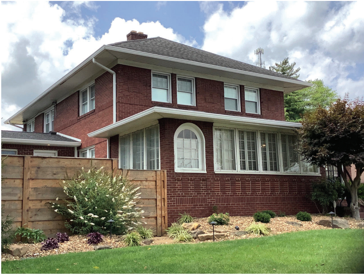
Photo ID 3103, House, 616 N. Main Street, Huntingburg; Alternative R
