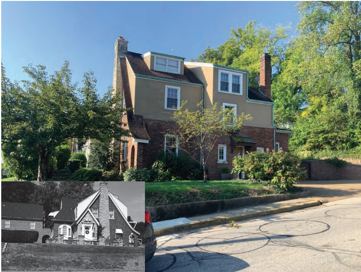
Photo ID 1970, Jasper Residential Historic District #2, potentially NRHP-eligible, 1445 Newton Street, Jasper; Local Improvement 4
