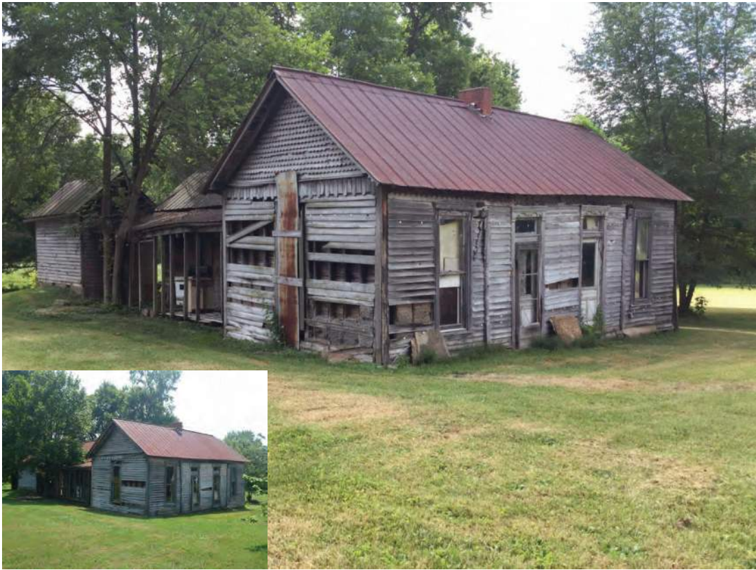
Photo ID 643, Chandler House, potentially NRHP-eligible, 6577 S Short Street, Alfordsville; Alternative C
