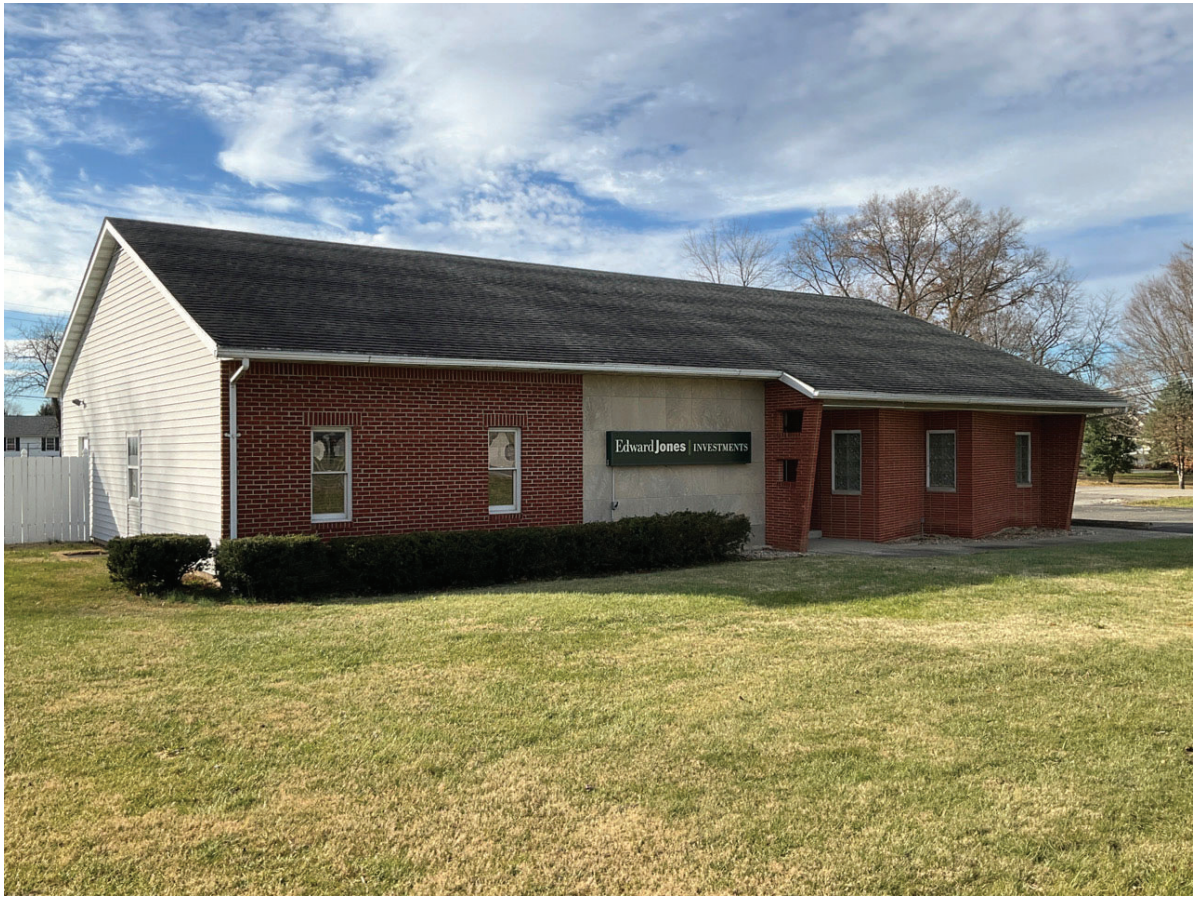
Photo ID 2177, Commercial Building, 402 W. Williams Street, Loogootee; Alternative P2
