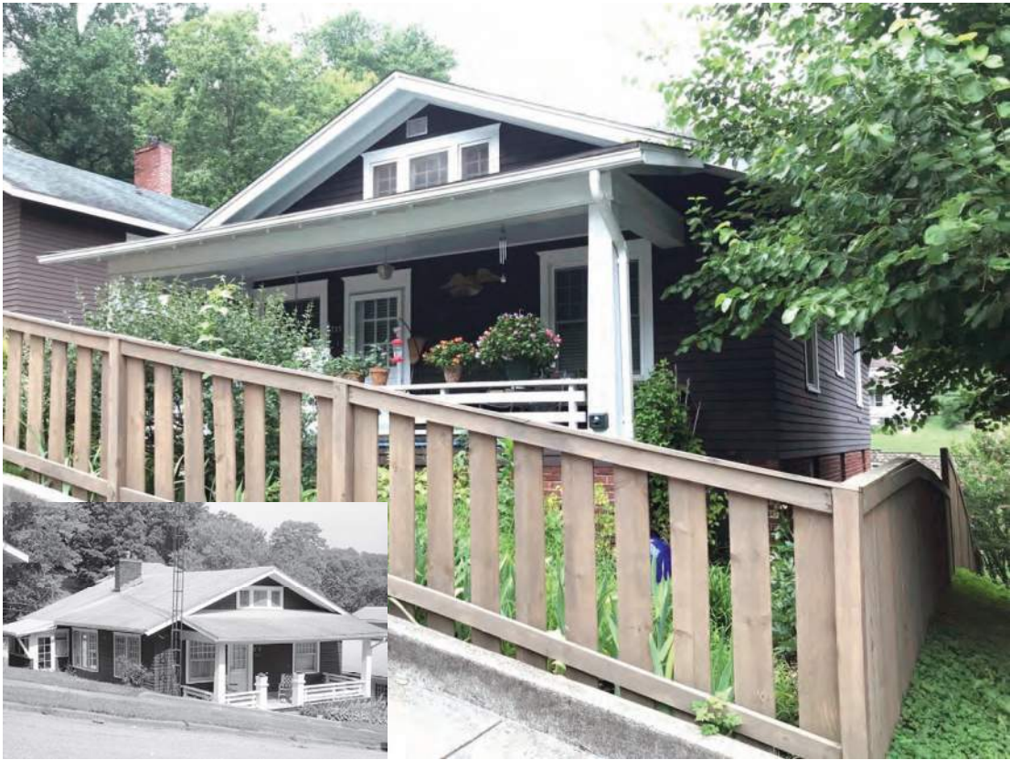
Photo ID 949, House, Ballard Homes Historic District, potentially NRHP-eligible, French Lick; Alternative O
