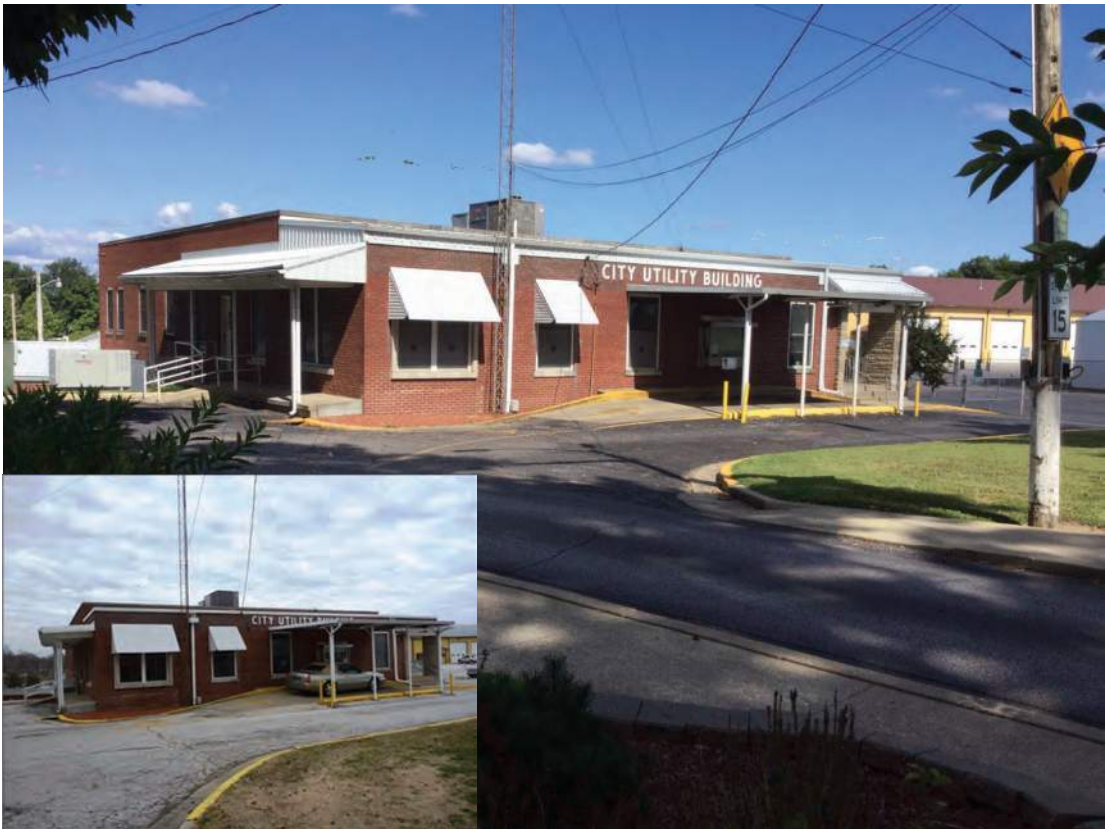
Photo ID 757, Utility Building, 2100 Memorial Avenue, Washington; Alternative C
