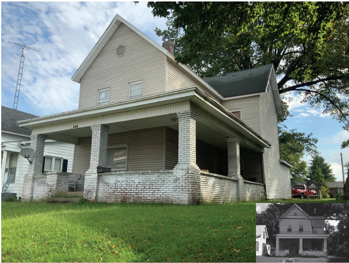
Photo ID 3170, House, Huntingburg Residential Historic District, 411 N. Main Street, Huntingburg; Alternative R
