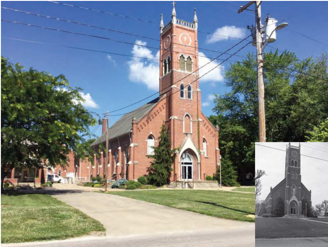
Photo ID 192, Saint Mary's Catholic Church, potentially NRHP-eligible, 2829 N 500 W, Ireland; Alternative C
