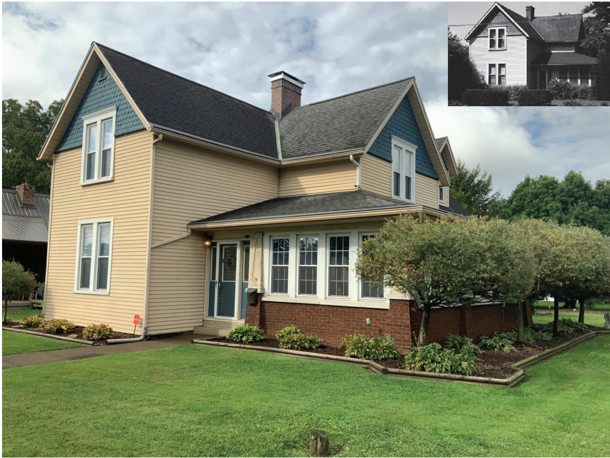
Photo ID 3145, House, Huntingburg Residential Historic District, 116 N. Main Street, Huntingburg; Alternative R
