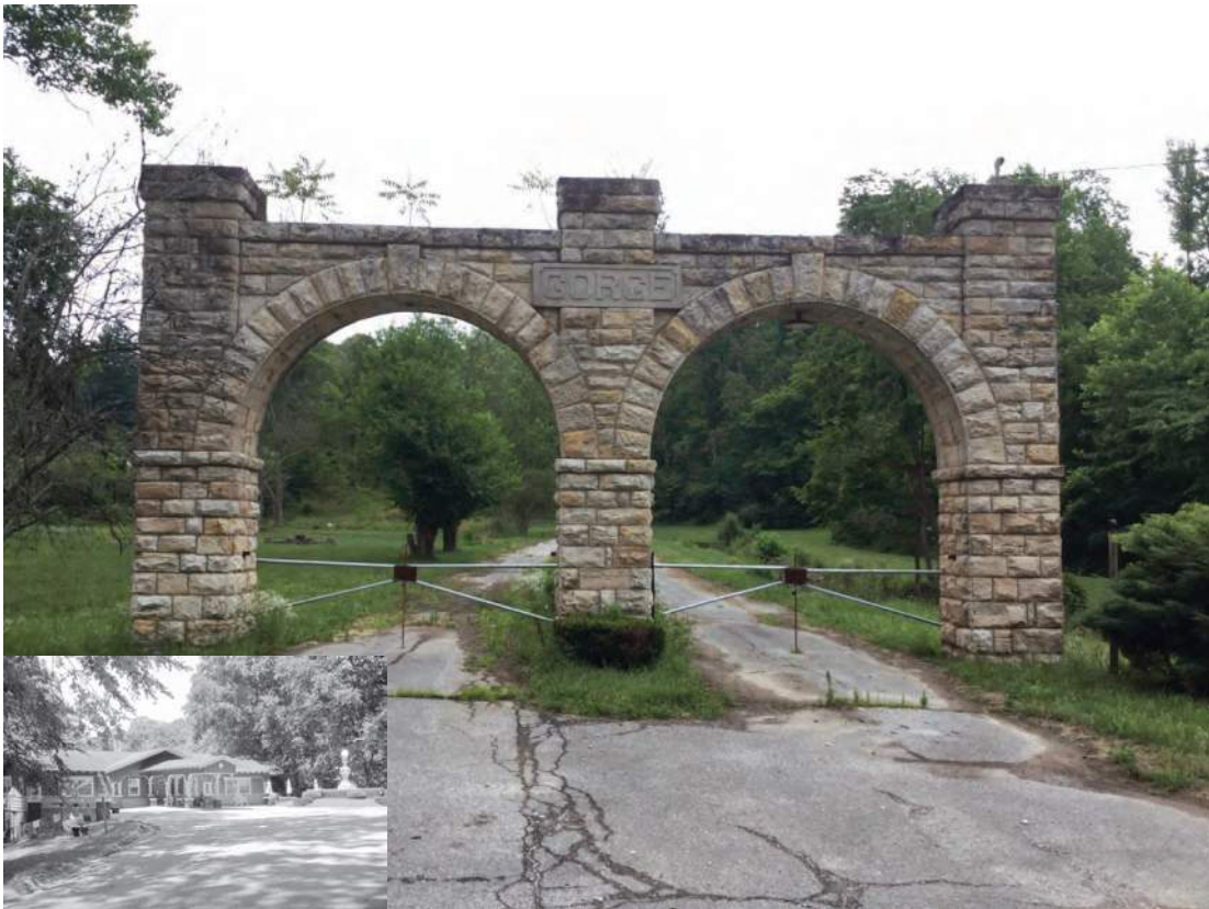
Photo ID 883, The Gorge Inn (entry), potentially NRHP-eligible, 6962 W. 175 S, Orange Co.; Alternative O
