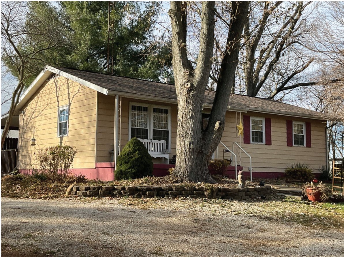
Photo ID 2184, House, 707 John F. Kennedy Avenue, Loogootee; Alternative P2
