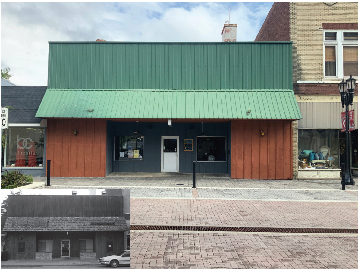
Photo ID 3156, Commercial Building, Huntingburg Commercial Historic District, 328 E. 4th Street, Huntingburg; Alternative R
