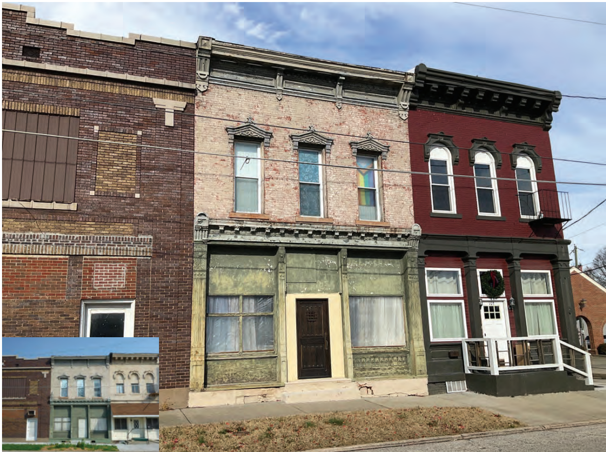
Photo ID 2152, Loogootee Commercial Historic District, NRHP-eligible, Commercial Building, 101 E. Main Street, Loogootee; Alternative P2
