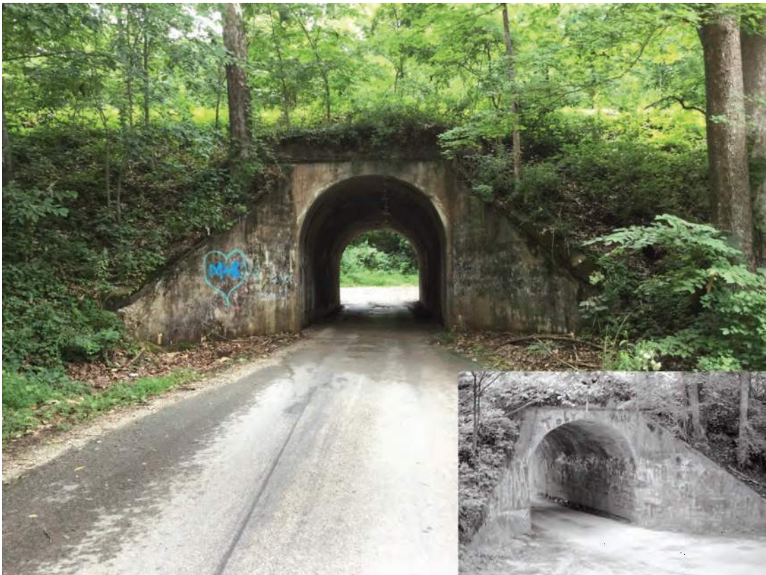
Photo ID 899, Southern Railroad Viaduct, CR 975 W, Orange Co.; Alternative O
