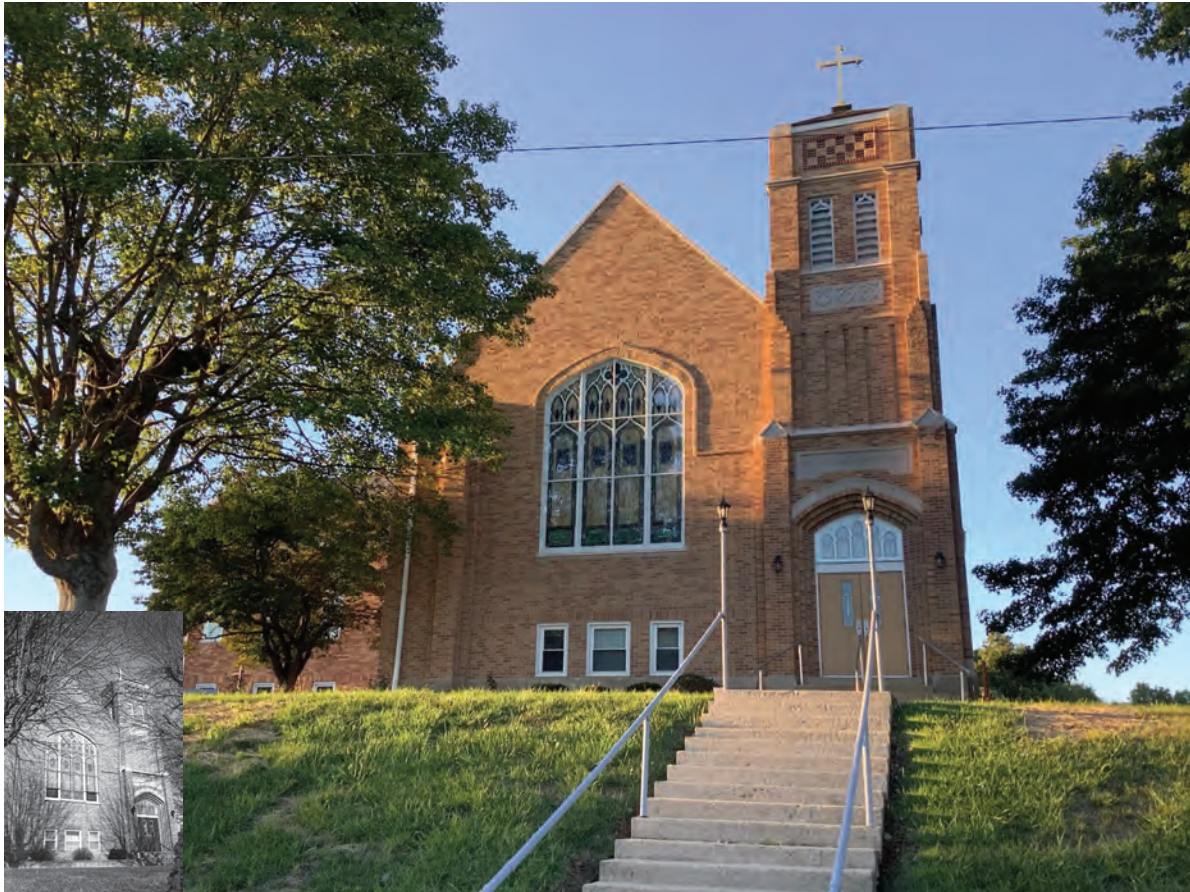
Photo ID 2104, St. John's Evangelical Lutheran Church, potentially NRHP-eligible, 5015 E. SR 56, Dubois Crossroads; Local Improvement 15
