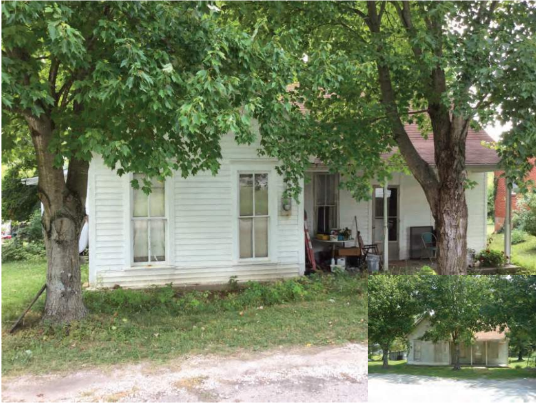
Photo ID 635, House, potentially NRHP-eligible, 6637 S. Main Street, Alfordsville; Alternative C
