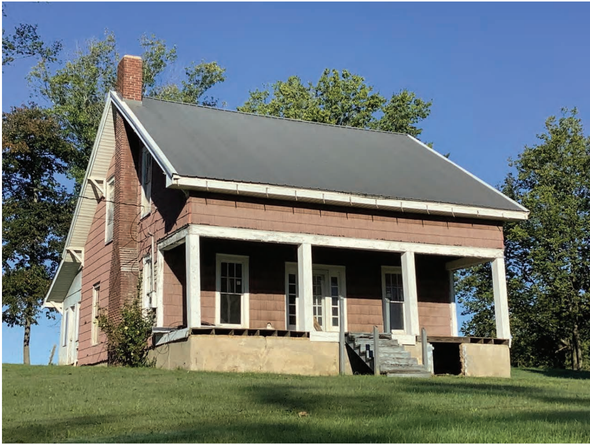
Photo ID 2087, House, 1748 Upper Sand Hill Road, Prospect; Local Improvement 18
