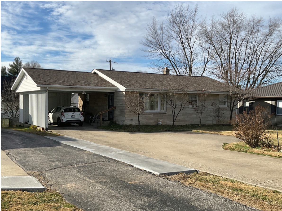
Photo ID 2173, House, 607 John F. Kennedy Avenue, Loogootee; Alternative P2
