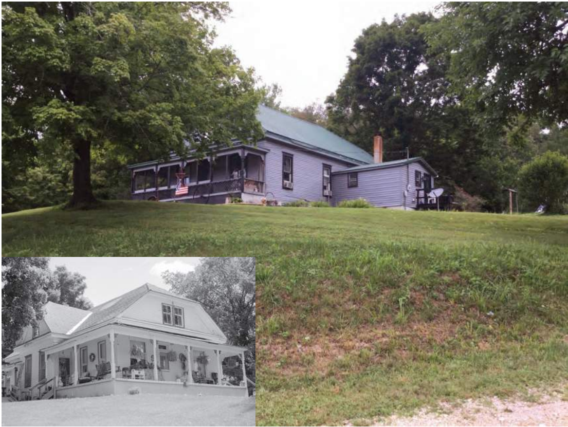
Photo ID 884, House, potentially NRHP-eligible, 7274 Gorge Road, Orange Co.; Alternative C
