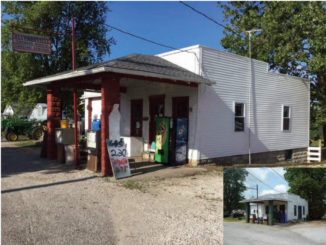
Photo ID 622, Tangbress Filing Station, potentially NRHP-eligible, 6422 Church Street, Alfordsville; Alternative C
