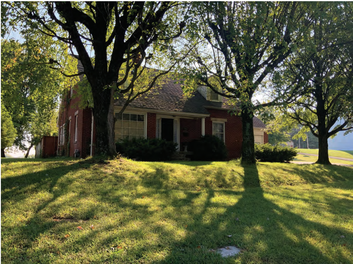
Photo ID 1994, Jasper Residential Historic District #3, potentially NRHP-eligible, 1732 Newton Street, Jasper; Local Improvement 4
