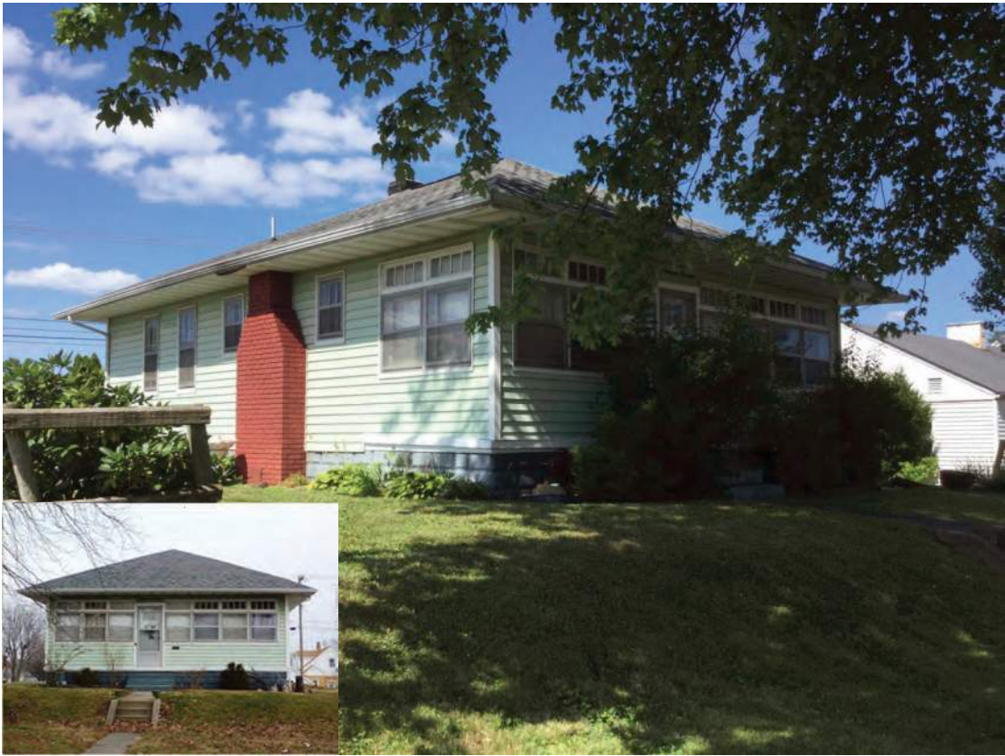
Photo ID 740, House, 1900 Memorial Avenue, Washington; Alternative C
