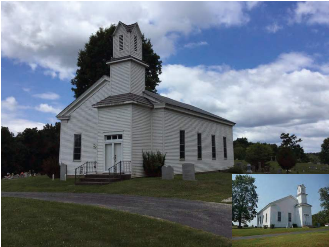
Photo ID 657, Old Union Church and Cemetery also known as Sugar Creek Church, NRHP-listed, CR 1125 Daviess Co.; Alternative C
