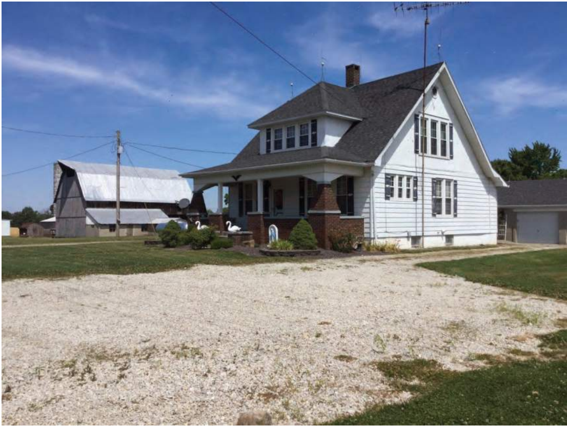
Photo ID 144, House, 4241 W. Division Road, Dubois Co.; Alternatives B, C
