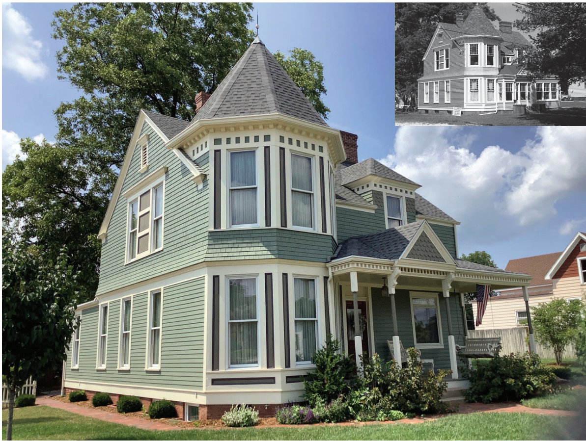
Photo ID 3106, House, Huntingburg Residential Historic District, 216 N. Main Street, Huntingburg; Alternative R
