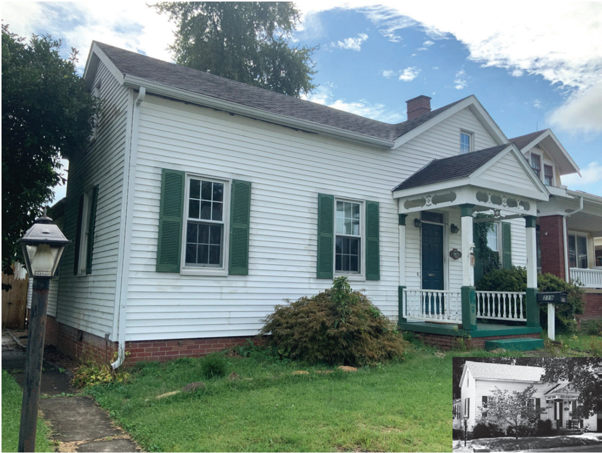
Photo ID 3176, House, Huntingburg Residential Historic District, 219 N. Main Street, Huntingburg; Alternative R
