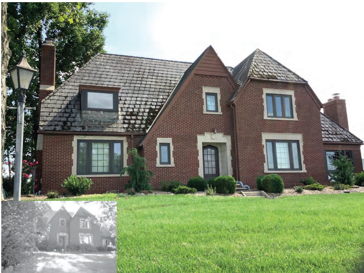
Photo ID 2113, Jasper Residential Historic District #1, potentially NRHP-eligible, 515 W. 6th Street, Jasper; Local Improvement 4
