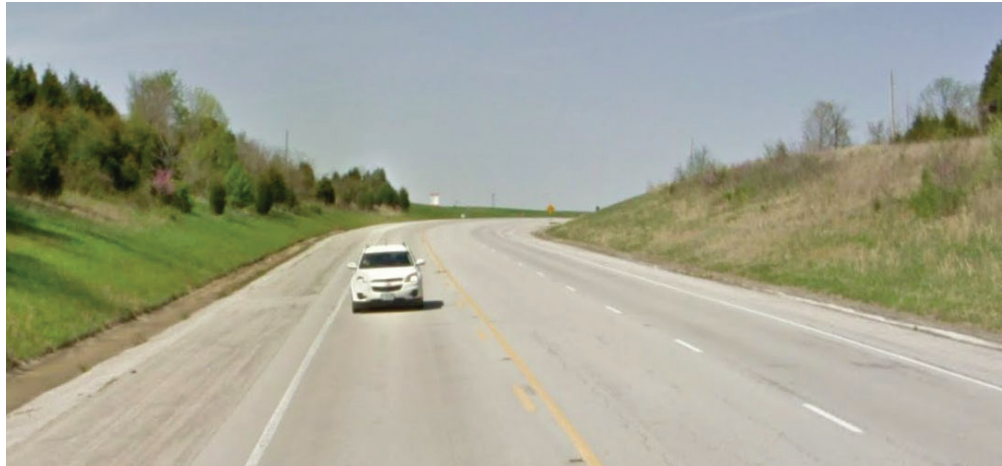
SR 145 in Crawford County
