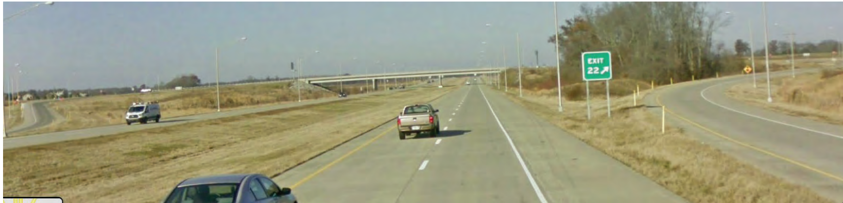
Interstate 69 in Gibson County
