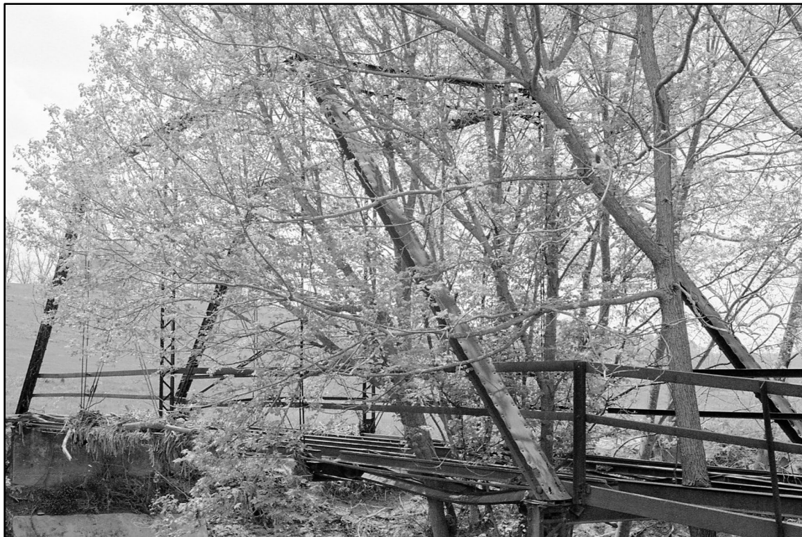
FIGURE 29. ORANGE COUNTY BRIDGE NUMBER 21 PHOTOGRAPH (c. 2005)
