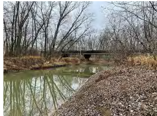
Figure 15. West side of US 231 bridge from south bank of Patoka River
