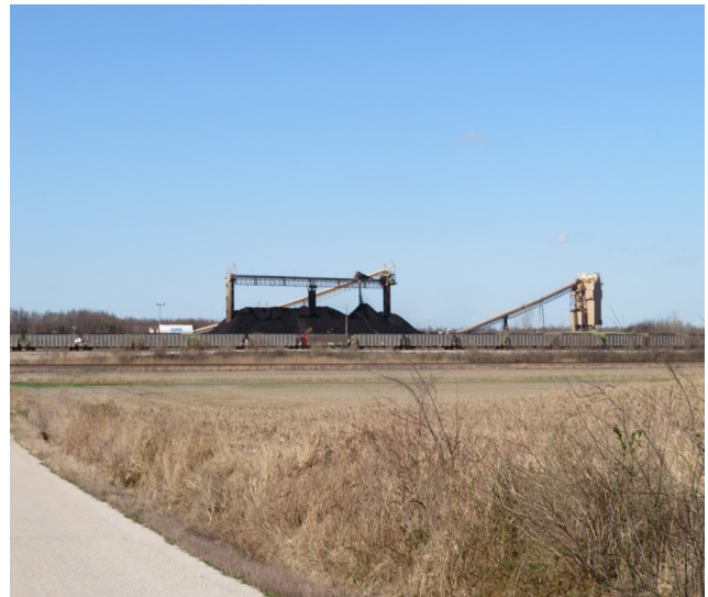
Figure 3.22-1: Coal Preparation Plant at an Underground Mine in Gibson County
