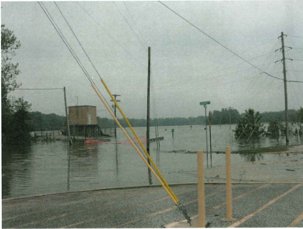
High Water 2011_05-08 on Kellerville Rd (Cathy Lane/Cherry St. Intersection area)
